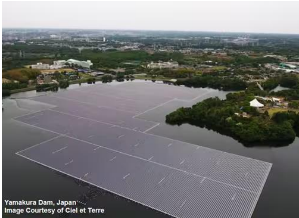
Figure 1. Floating solar at Yamakura Dam, Japan
